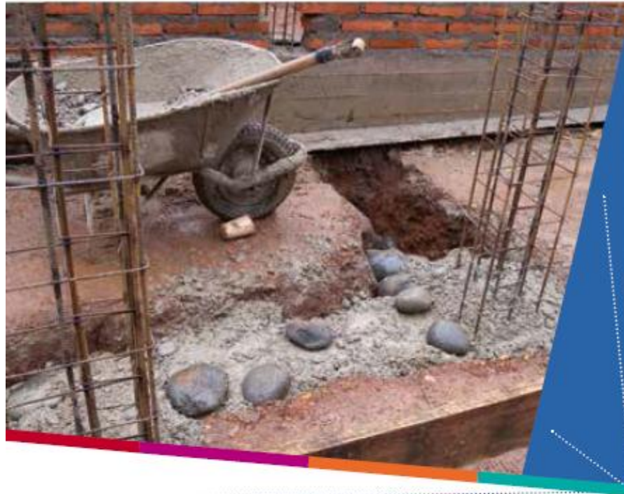
Image 1: Tie-column reinforcement cages extending from foundations of a new building; these are a key feature of 'confined masonry' construction. Source: Brzev, Astroza and Yadlin, 2010 1 .
